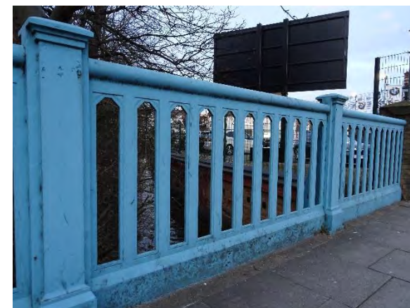
Bridge over River Quaggy, Lee High Road
