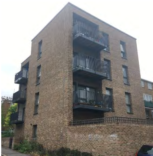
New Homes, Lee Church Street
