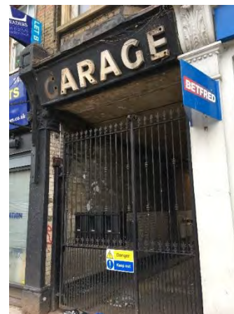
Old Garage Entrance, Lee High Road
