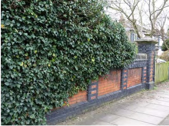
Bridge, Manor Park
