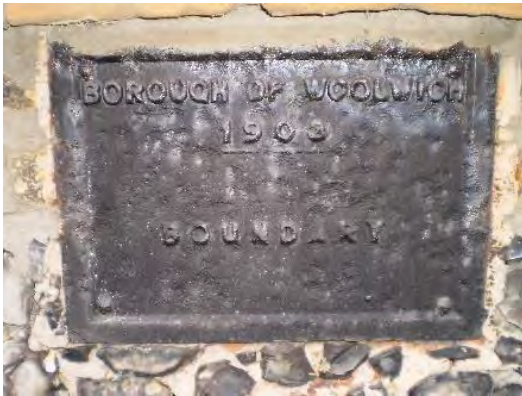
Boundary Marker (1903) on the east parapet of the bridge taking Weigall Road over the Quaggy
