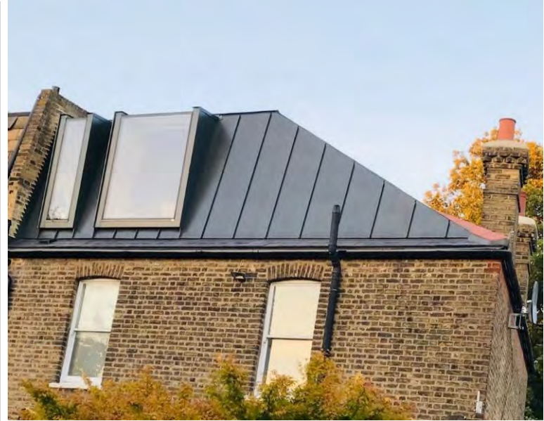
Right: Lee Forum area/ This loft extension has minimal visual impact on the view from Manor House Gardens, or on the perception of the original roof form. It is also clearly read as an early twentieth century addition to the original house, using modern materials and glazing forms. Neel Dakshy Architects
