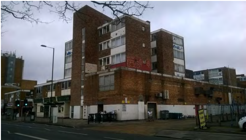
Leigate, Burnt Ash Road
