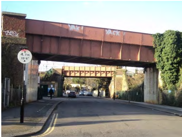
Two railway bridges at Manor Lane
