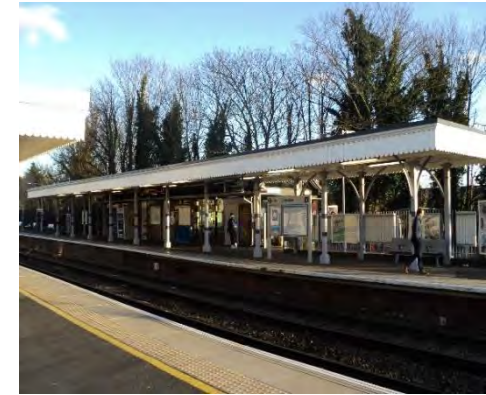
Platform 1, Lee Railway Station
