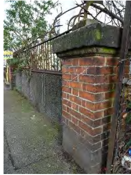
Bridge, Eastdown Park
