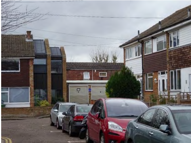
Left. Wolfram Close, Lee Forum area. The staggered forms of this two storey extension and change of materials distinguish it from the original building. Details like the cast concrete pads and gutter zinc gives a streamlined finish. The 2 sections of the recessed extension, set back from the public realm, do not intrude on the eye or the surrounding space and nearby dwellings, but blend in. The development allows for small front garden spaces and synchronicity with the original house. Selencky /// Parsons Architects
