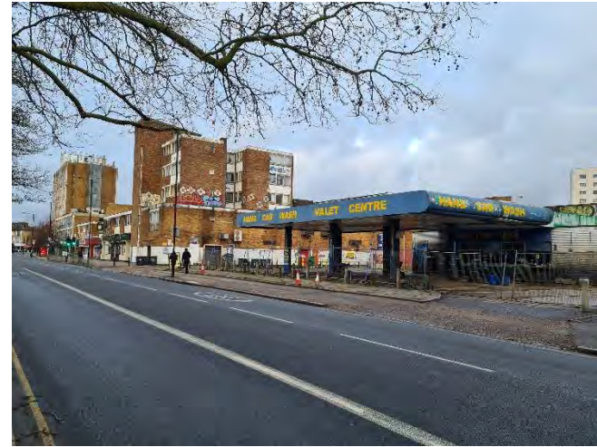
Leegate Shopping Centre, SA10
